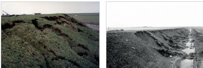
Figure 7: Slope parallel sliding.
