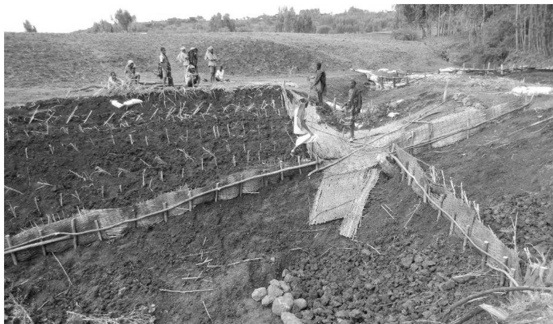
Figure 7. Construction of gully erosion control measure in the Debre-Mewi watershed, Ethiopia. Erosion control consists of regrading the gully head cut and sidewalls to approximately 40-45 degrees and protecting the soil surface with bamboo sheets and vegetation.
