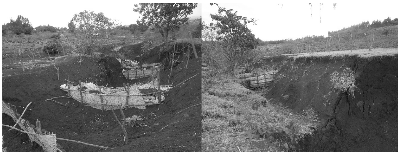
Figure 1. Check dams in the Debre-Mewi watershed, Ethiopia. Left: newly constructed check dams to stabilize a gully. Right: gully head-cut migrating towards upstream check dams.
