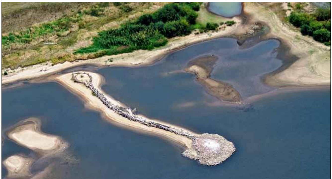
Bild 13: Bühne 23a El-km 450,55 linkes Ufer / 2009 Figure 13: Groyne 23a, Elbe kilometer 450.55, left bank / aerial photograph dated 2009
