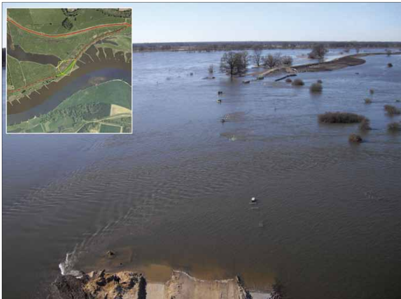
Bild 3: Altdeichschlitz 1 (Position 1) Figure 3: Slot 1 made through the old dike (location 1.1)
