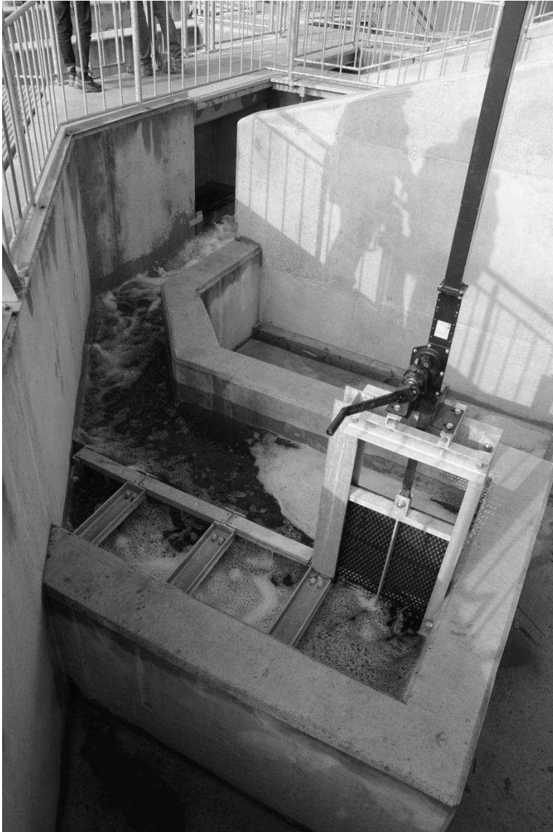
Figure 9. Monitoring station for fishes migrating downstream through the surface bypasses.
