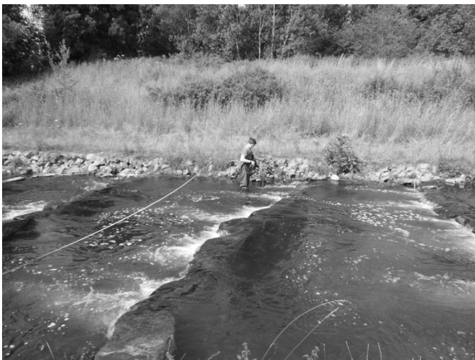
Figure 9. Full cross-bar block ramp, Brückerbach, upstream part.
