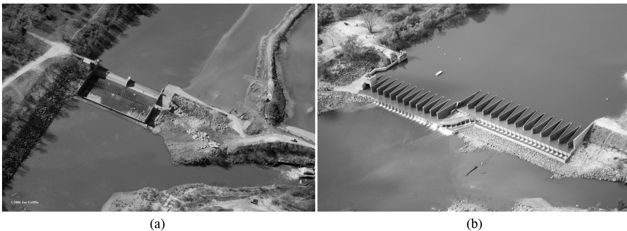
Figure 1. Brazos Dam (a) before the spillway upgrade [crest-gated spillway (left) and emergency embankment spillway just after demolition started (right)] and (b) after the spillway upgrade project (two-segment labyrinth weir) (photos courtesy of the City of Waco, TX, USA).
