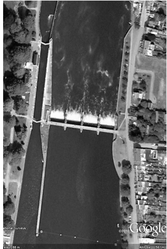
Figure 5. View of the La Plante dam (GoogleEarth)
