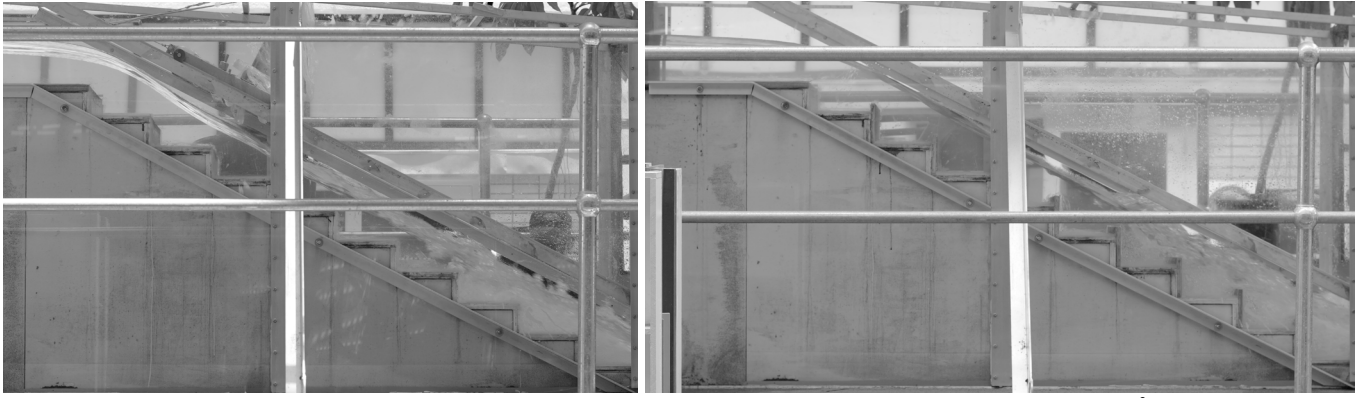
Figure 3. Skimming flow regime on flat and pooled stepped spillways - Left: flat steps, Q = 0.114 \text{ m}^3/\text{s} , d_c/h = 1.7 , Re = 8.8 \times 10^5 ; Right: pooled steps, Q = 0.100 \text{ m}^3/\text{s} , d_c/h = 1.56 , Re = 7.7 \times 10^5
