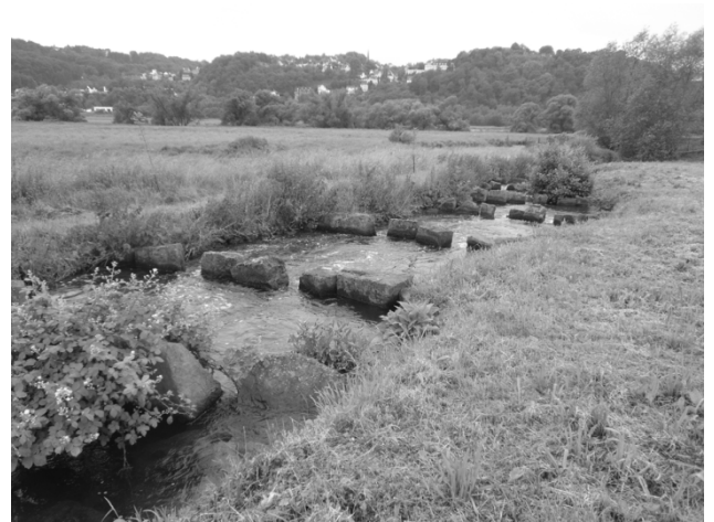
Figure 8. Bypass cross-bar block ramp Harkort reservoir, upstream ramp part.
