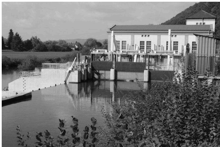
Figure 1. Unkelmühle/Sieg Hydroelectric Plant with new upstream bar screens, view from the upstream side.
