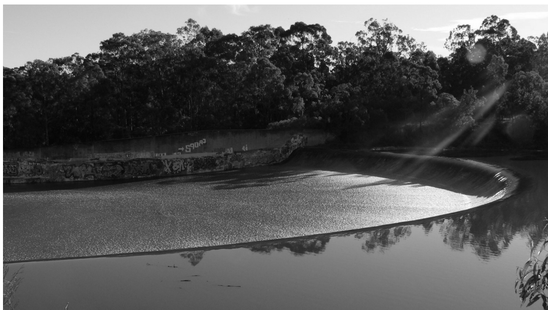
Figure 5. Inlet of the minimum energy loss (MEL) weir spillway of Lake Kurwongbah (Petrie QLD, Australia) on 22 May 2009 during a small overflow
