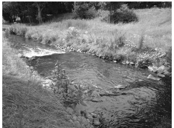
Figure 10. Full cross-bar block ramp, Brückerbach, downstream part.
