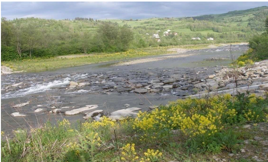
Figure 1. Studied rapid hydraulic structure (RHS) in Porębianka Stream
