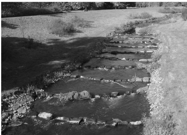
Figure 4. Cross-bar block ramp (River Brückerbach, Düsseldorf, Germany).
