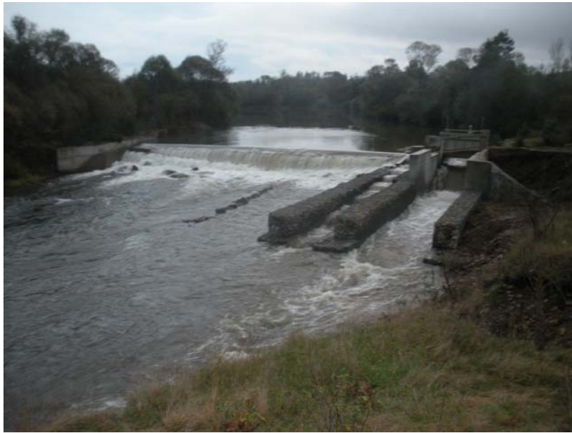
Figure 3 Installation site view after reconstruction of the existing facilities
