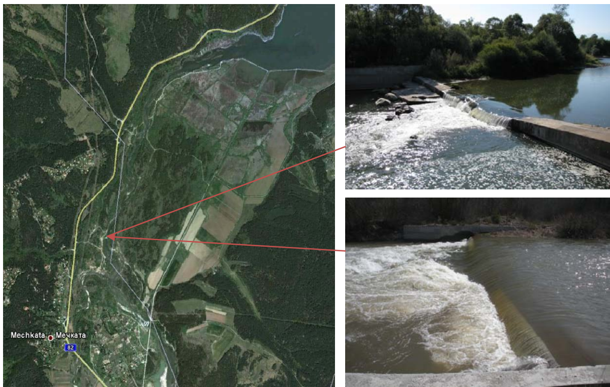
Figure 1 Installation site at River Iskar and photographs of the existing sill under different flow conditions.
