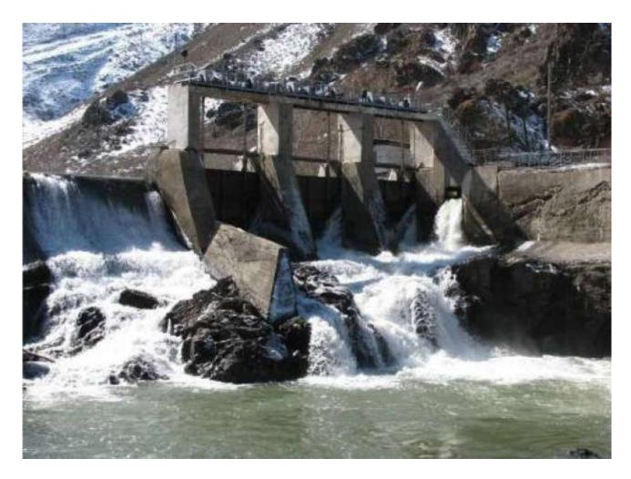
Kyzylagash (Kazakstan) dam breached by overtopping (2010)
