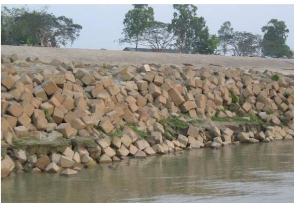
**Fig.6** Steep cohesive banks cannot be covered with falling aprons
